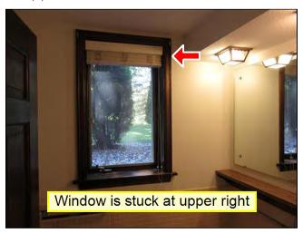
**10.6** (5) Loose cranks at 2nd floor northwest bedroom need to be tightened.
