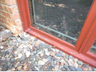
**2.4** (2) Noted some basement widows have sills sitting right at grade level. This is problematical over time because the wood soaks up moisture from the ground it is in contact with. Keep good paint coverage to preserve the life of the wood. Also see comments in Grading section.
