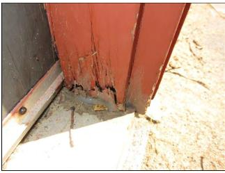
2.0 (2) Some decayed trim noted. Repair any soft wood as needed. Overall condition of the trim is good.
