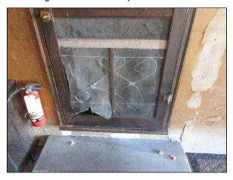
**3.6** (1) Loose threshold needs to be secured.
